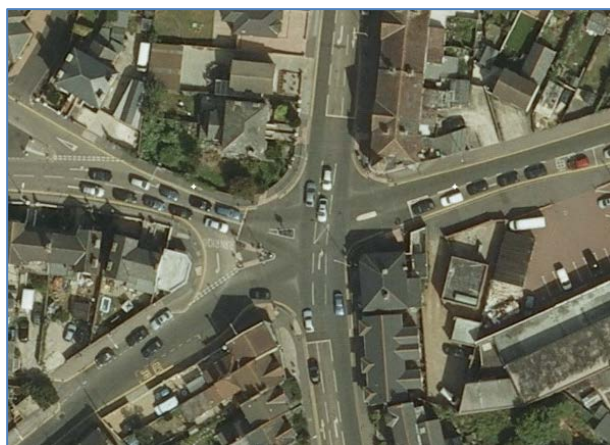
Figure 18 – Victoria Traffic Signals
